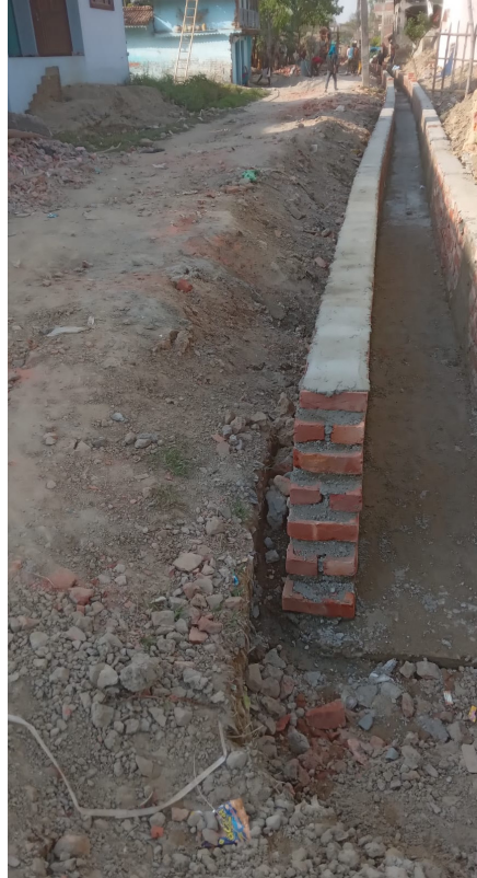
Home connected to covered drainage system (above); drainage under construction (right).
